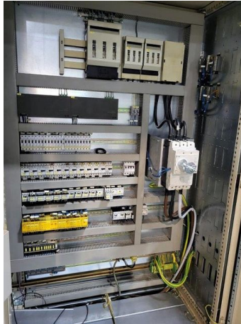
E Cabinet Inside
